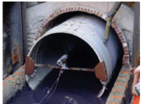
Conventional slip-lining of non-circular pipes results in a large annular space & loss of flow capacity; these are just a few of the problems that will be eliminated when StifPipe™ is used!
