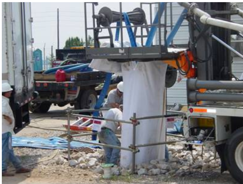
Figure 2-2 Water-Filled Liner at Launching Point
