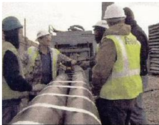
Figure E-3 Strapped PE Pipe Ready for Insertion
