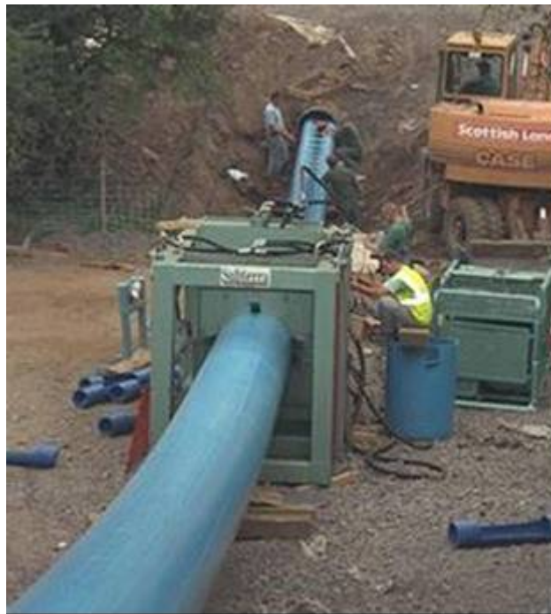
Figure E-2 PE Liner Pulled Through Former
