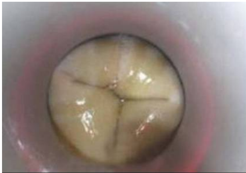
Figure 2-4 Inverted Liner Progresses as it Unfolds in Host Pipe
